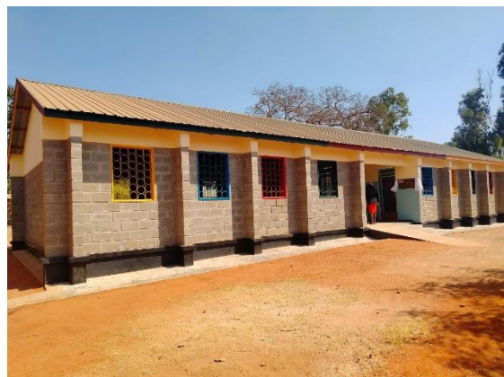
Newly constructed classroom block
