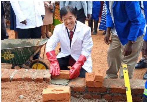
(Left) Ambassador Iwakiri laying foundation stones (Right) Ambassador giving a speech
